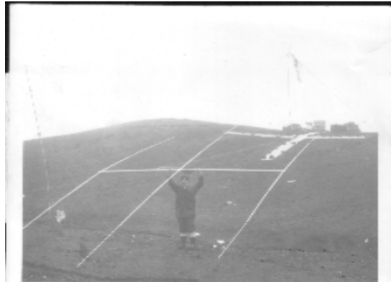
The 20M beam ready to go up. The cross on the hillock behind is a survey marker. The 36ft vertical is sited here too.
