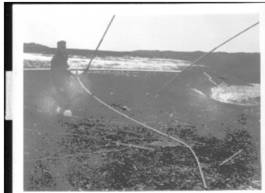
What goes up..... Just after the mast collapsed.
